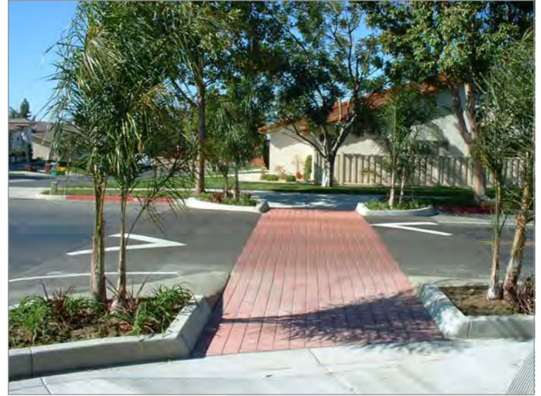
An example of a crosswalk that is both raised and made of materials different from the rest of the street. Two goals of these features is to make drivers more aware of crosswalks and to slow traffic down.
