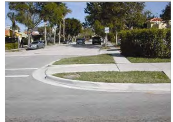
An example of a bulbout on a neighborhood street. Bulbouts are designed to reduce the distance pedestrians must walk to cross streets and to make them more visible to passing cars.
